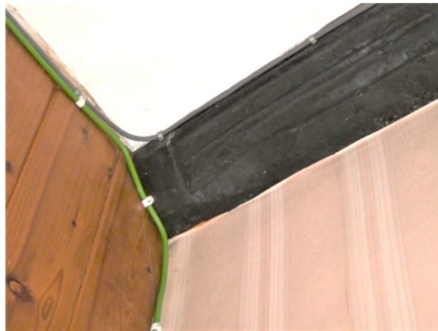
Figure 26: Double ovolo cross beam on the sitting room side of the entrance hall
