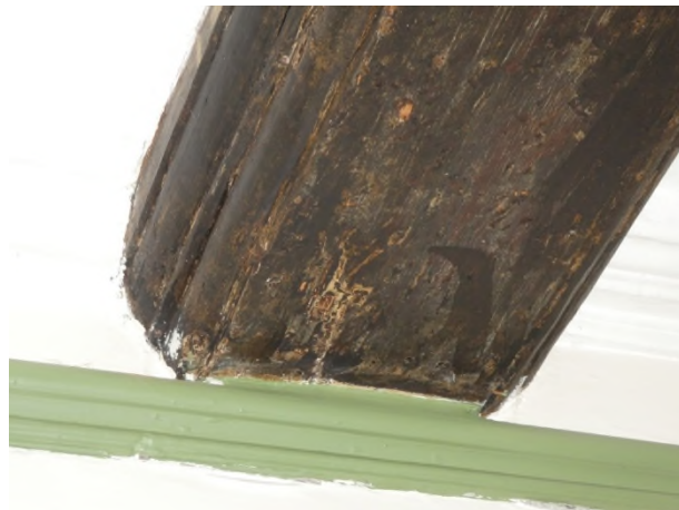
Figure 21: Detail of the double ovolo axial beam
