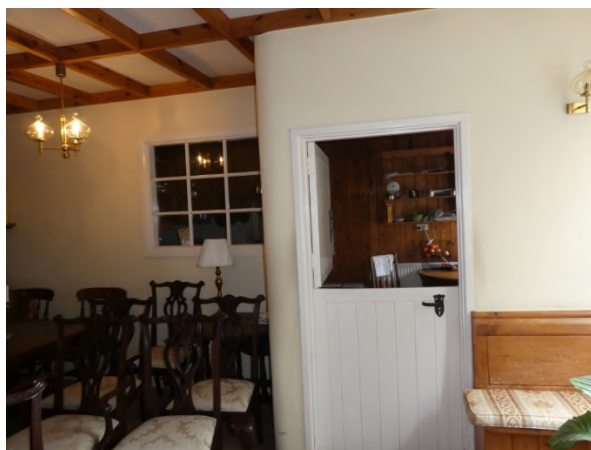
Figure 24: 20 th century partitions in the dining room/kitchen
