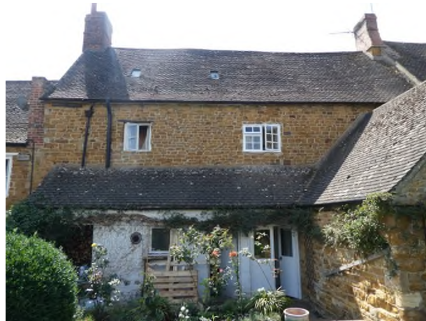
Figure 20: Rear elevation of Phase 2
