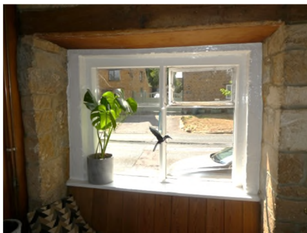
Figure 54: Late 19 th century window in an earlier frame in the kitchen
