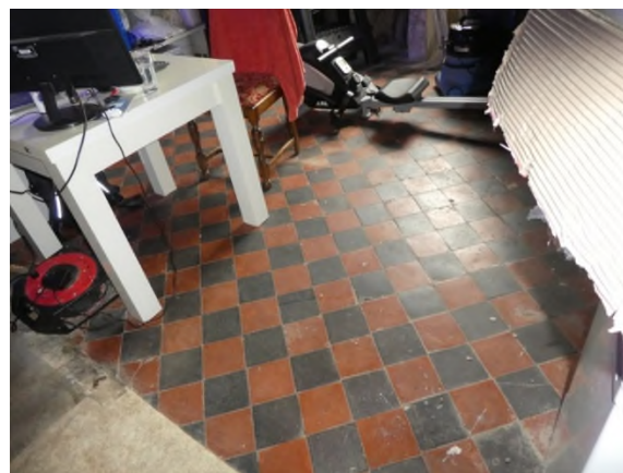
Figure 61: Tiled floor in the workshop
