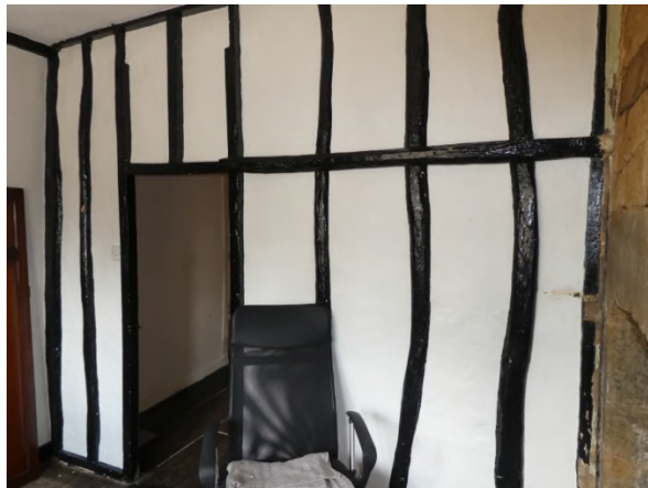
Figure 57: Stud partition between bedroom 3 and the bathroom
