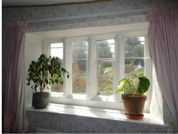
Figure 38: Plain chamfered mullion window in bedroom 2
