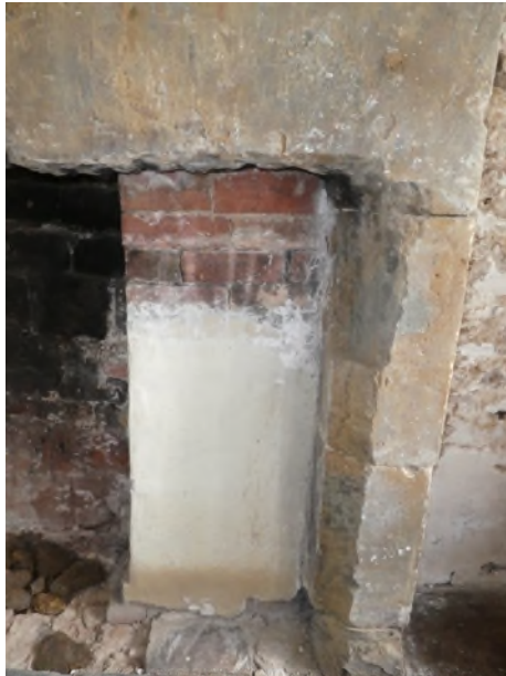
Figure 58: Brick flue inserted into the 17 th century fireplace
