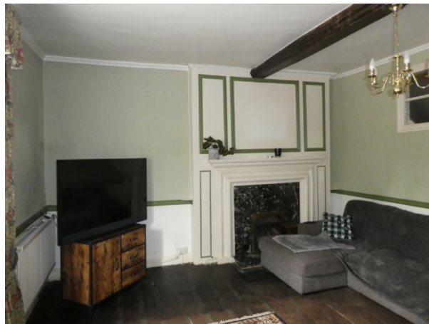
Figure 20: Axial beam and wide floor boards in the sitting room
