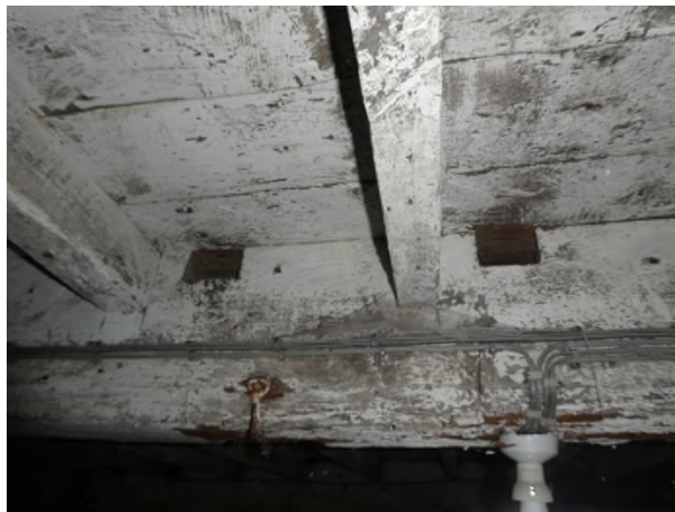
Figure 31: Detail showing mortises for the original joists
