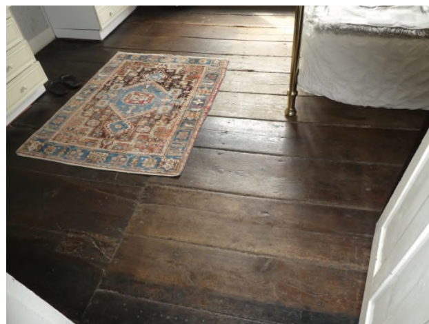
Figure 35: 12" wide floor boards in bedroom 1
