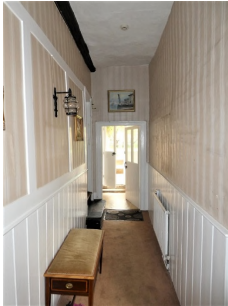
Figure 25: Entrance hall looking towards the rear door (note the double ovolo cross beam to the left)
