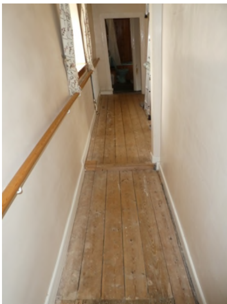
Figure 40: Narrower boards and a step up in the passage leading to bedroom 2 and the bathroom/bedroom 3
