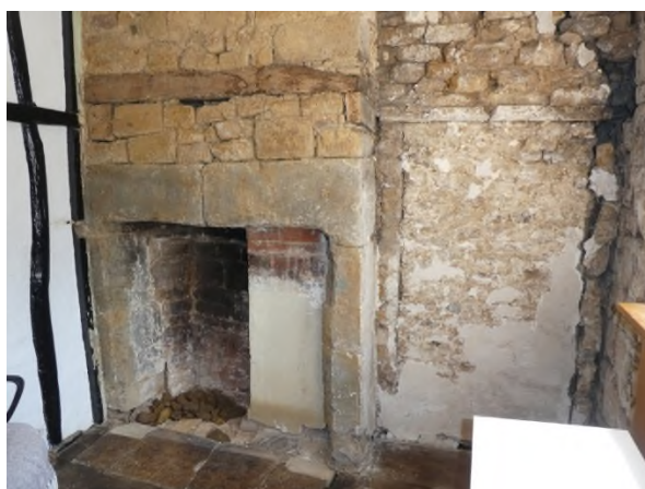
Figure 41: Stone fireplace and blocked door on the south-east side of bedroom 3
