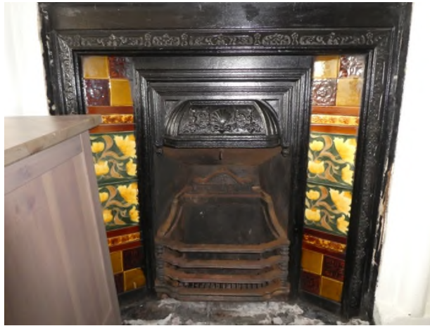
Figure 56: Late 19 th century register grate in bedroom 1
