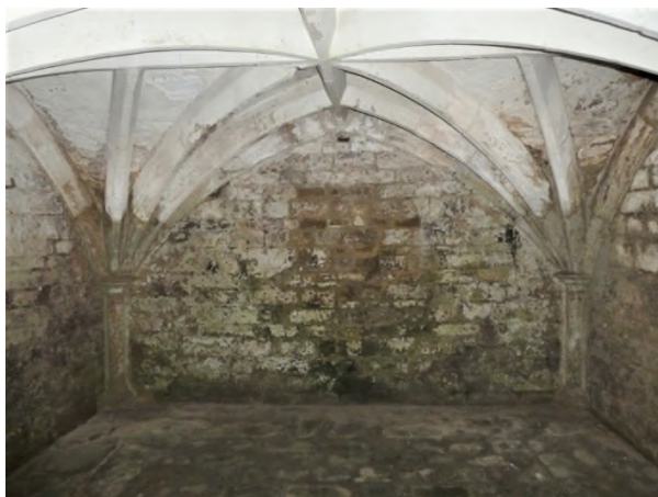
Figure 10: Rear wall of the cellar
