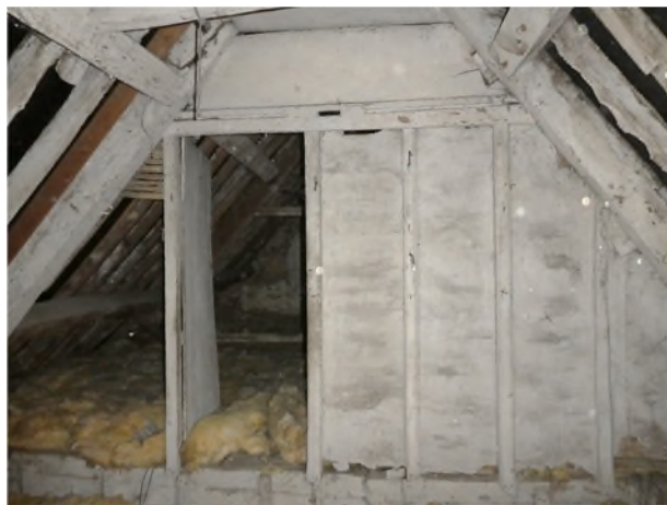
Figure 45: Stud partition on the north-west side of the central bay
