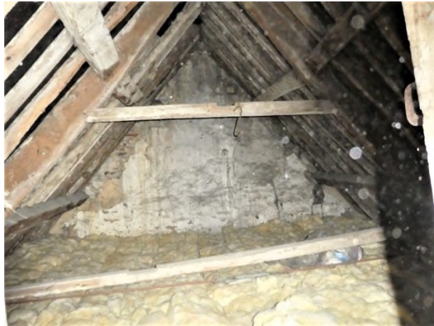
Figure 44: Butt purlin roof structure
