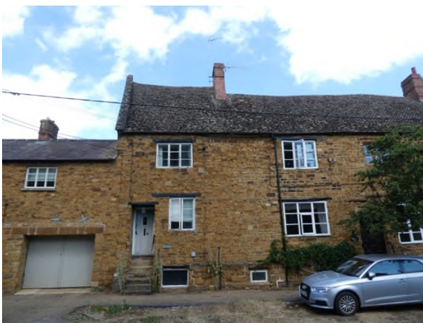
Figure 17: Window openings with timber lintels on the left hand side of the front elevation
