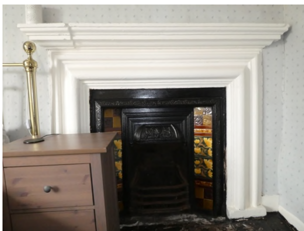
Figure 48: Early 18 th century bolection fireplace in bedroom 1
