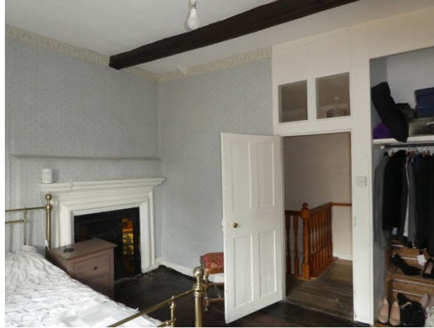
Figure 33: Axial beam with double ovolo mouldings in bedroom 1
