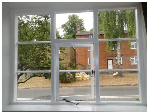
Figure 59: 20 th century replacement window – sitting room
