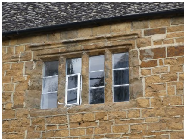
Figure 15: First floor stone mullioned window with hood mould
