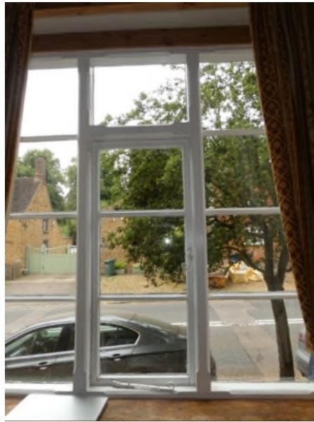
Figure 59: 20 th century replacement window – dining room
