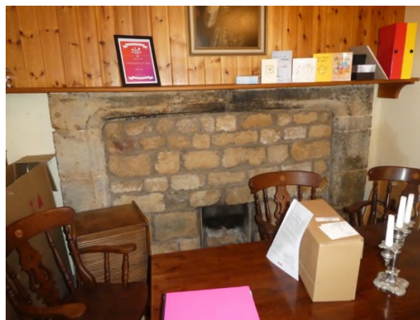
Figure 23: Detail of the fireplace in the dining room
