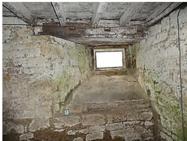
Figure 32: Splayed opening with slope and lintel with mortises for joists
