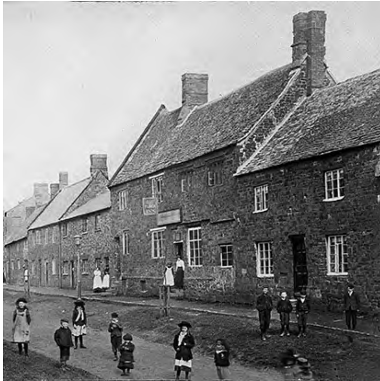
Figure 5: Photograph of Plough House in c. 1905
