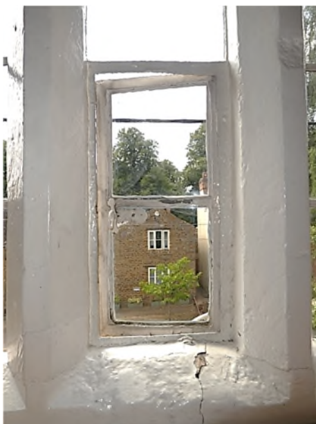
Figure 43: Detail of the iron casement with catch and decorative back plate
