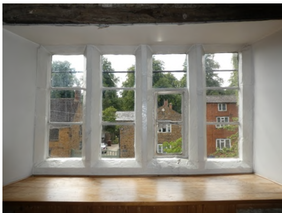
Figure 42: Plain chamfered mullion window on the south-west side of bedroom 3
