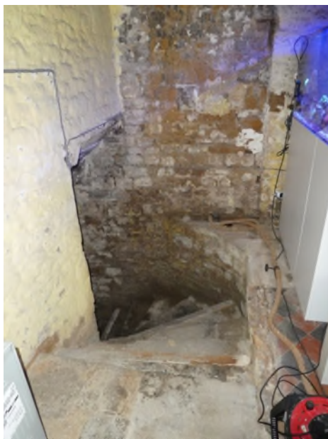
Figure 27: Entrance to the cellar from the workshop
