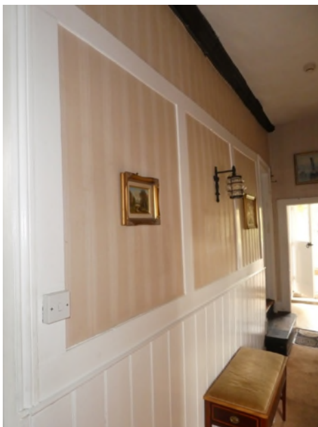
Figure 53: Late 19 th century matchboard dado with probably 20 th century applied boards above
