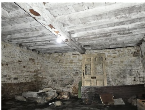
Figure 29: Axial beam and replacement joists in the cellar
