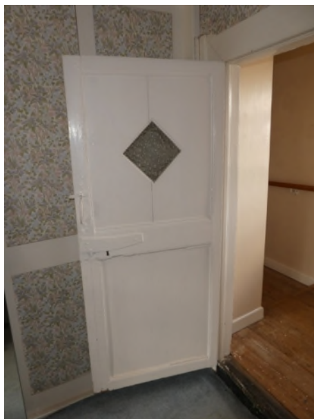
Figure 37: Late 17 th century 2-panelled door to bedroom 2
